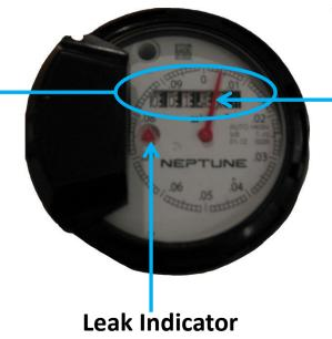
Movement of this triangle when all water fixtures in home are closed suggests a leak
