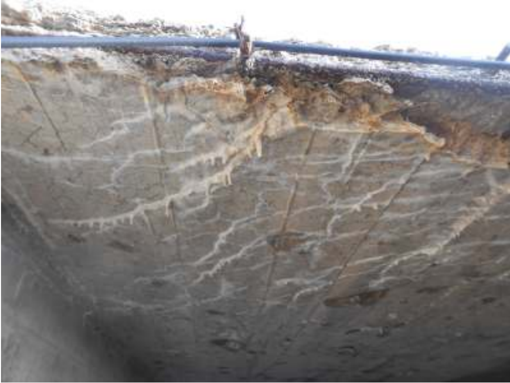
Photo 11: Soffit, west end
