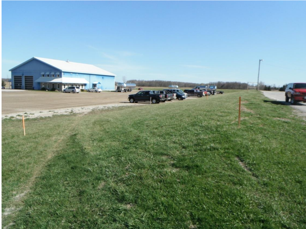
Plate 5: Disturbed Area, Not Assessed
