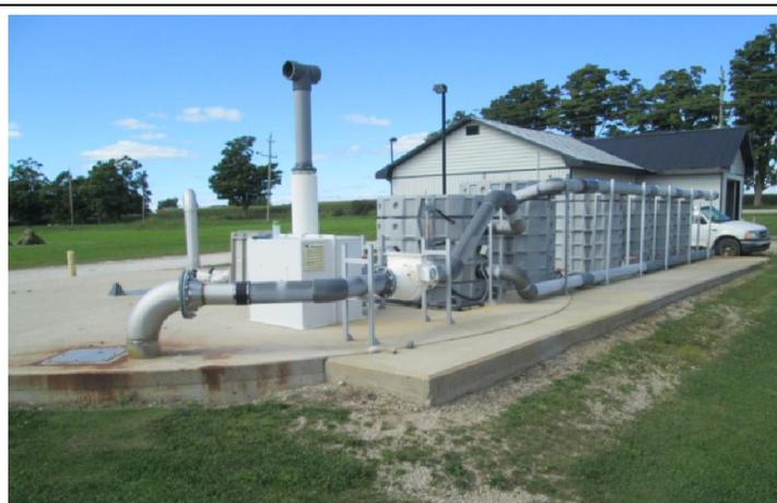
**Figure 1. Septage Receiving Station – Equalization Tank and Biofilter Odour Control Units**
