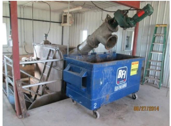
**Figure 4. Septage Receiving Station – Grinding/Screening Equipment**
