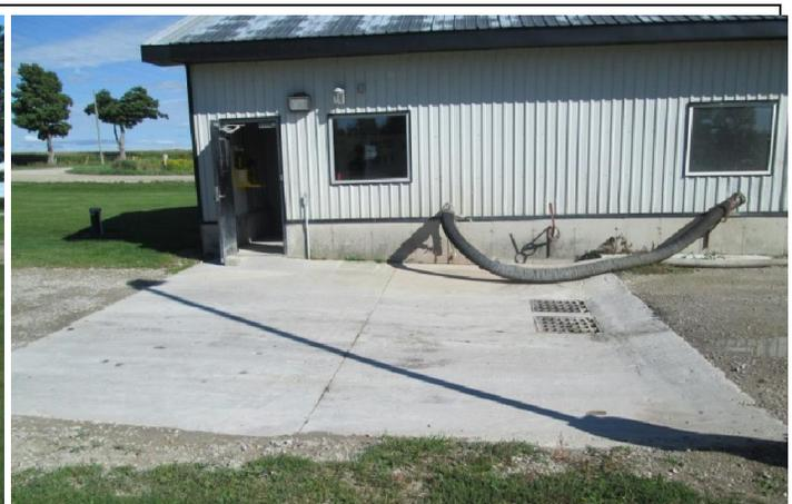
**Figure 2. Septage Receiving Station - Sewage Hauler Unloading Bay and Metering Station**
