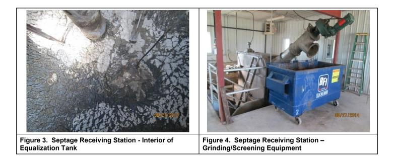
The overall objective of constructing the SRS was to reduce shock loading to the plant by storing high-strength hauled waste off-line temporarily, then metering it into the plant at a controlled rate. There is only 1 truck unloading connection (i.e. only 1 truck can unload at once). However, recent operating experience indicates that due to high use of the facility, the plant continues to experience occasional shock loads, although not as pronounced as before the facility was put into service.
