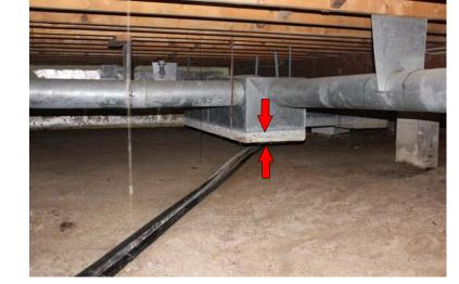
The large rectangular air plenum box in crawlspace is suspended directly below the main floor furnace. Staining and rusting at bottom 4" of plenum box records elevation of previous water accumulation in the crawlspace. Furnace air, flowing over uncontrolled water source, is a health concern.
