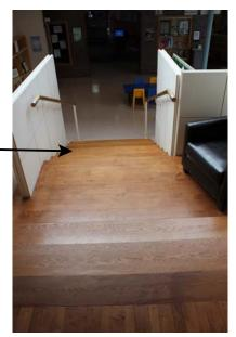
Nosings at interior stairs are not visibly distinguishable from flooring and treads, thus presenting a potential trip/stumbling condition.
