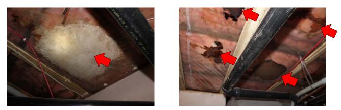
Suspect mould and water staining is visible on top of polyethylene vapour barrier, located above the suspended ceiling system, which is part of the insulated floor assembly between main and second floors. Roof leaks are the likely contributing factor, although, this could not be confirmed because the door to the second floor was secured.
