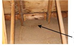
Water tracked down underside of sloped roof and eventually penetrated the building, causing damage.
