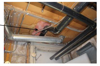
Openings in gypsum board ceiling, of north mechanical room, compromise the required fire-rating for the room.
